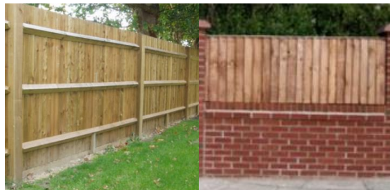
1.8m Close boarded timber fence and 1.8m brick wall with timber fence in fill.
